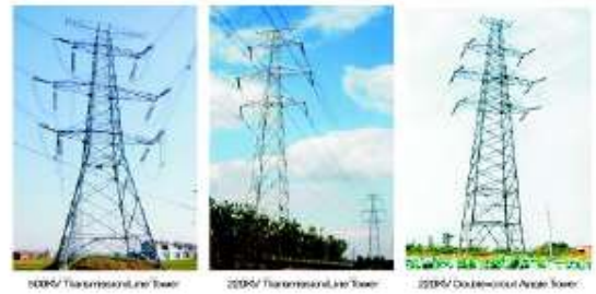
220kV Transmission Line Tower
