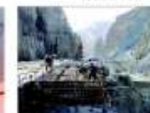
Shenyang Zhongyuan Tunnel of Great Mountain
