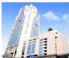
Shahin Shopping Mall Commercial Complex Car Parking System
