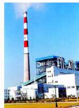
Changshu 300MW Thermal Power Plant, Jiangsu Province
