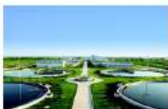
Yundong Sewage Treatment Plant, Chengde (with a treating capacity of 100,000 M3)
