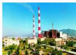
Hainan Hainan 4200MW Thermal Power Plant Hainan Province
