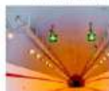
Shanyi Zhongyuan Tunnel of Great Mountain
