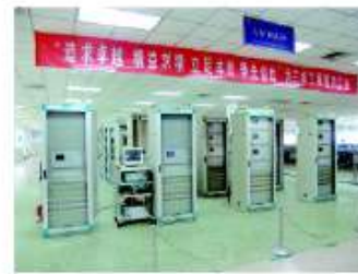
Micro-processor based protection relays and metering devices for three-phase power
