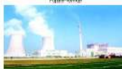
Jiangxi 1300MW Thermal Power Plant, Shandong Province
